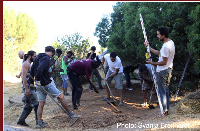
Building Swales in the Testfield and learning about rain water harvesting
